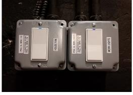
installed a remote switch at the end of the alley for the fan, as well, so there is still control of the fan outside of the booth. I also replaced the double Work Light switches at the end of the alley with a single switch, which controls both "banks" of Work Lights together for simplicity.
