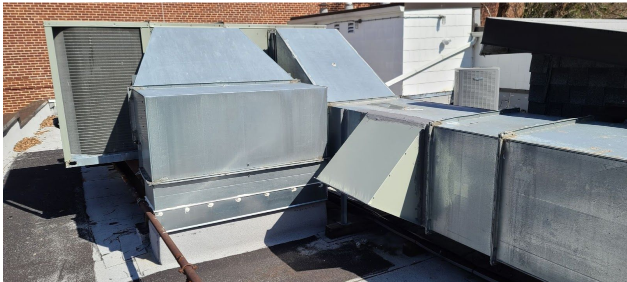
New fresh air intake on performance space HVAC
