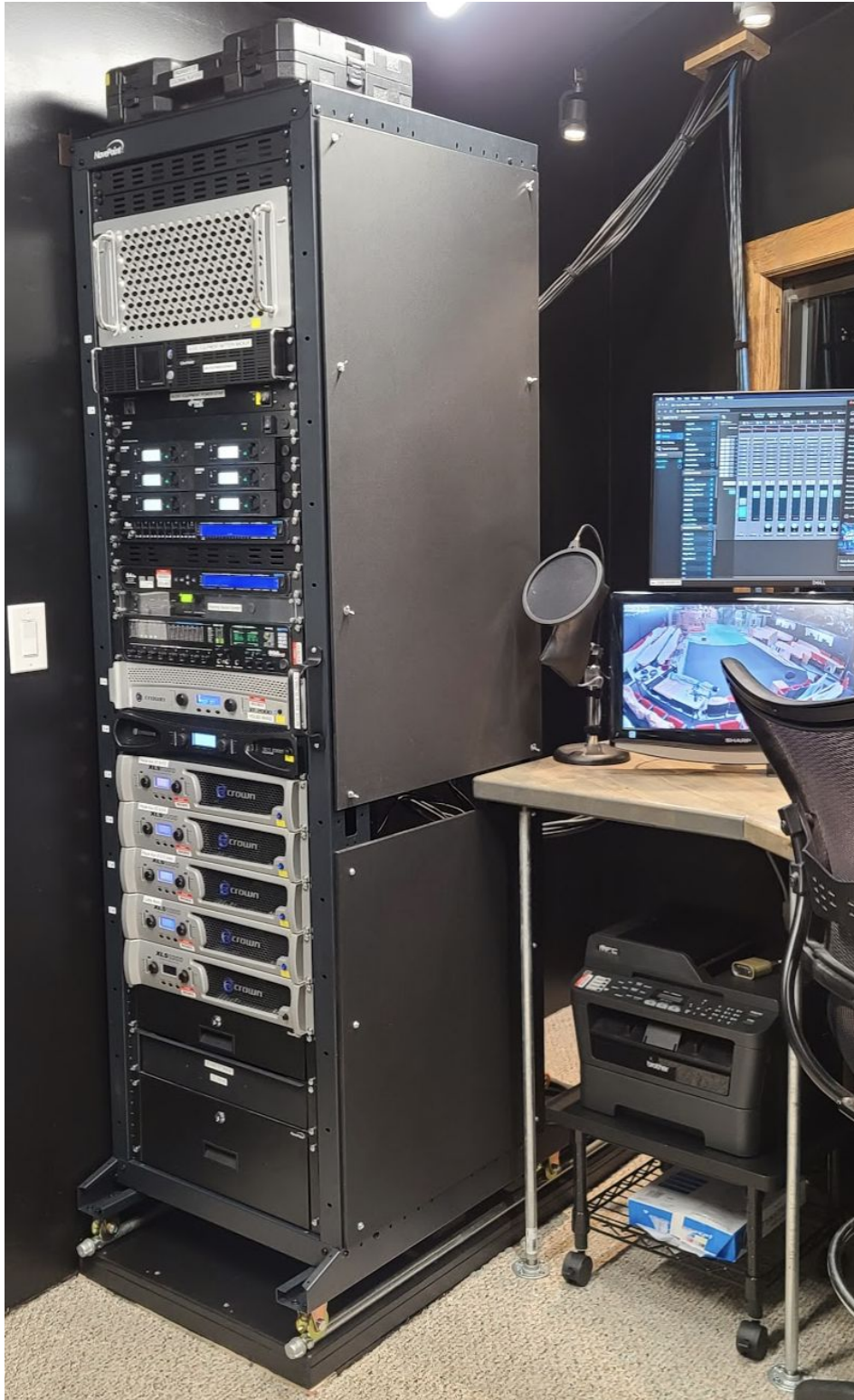
Sound rack shown rolled out to maintenance position
