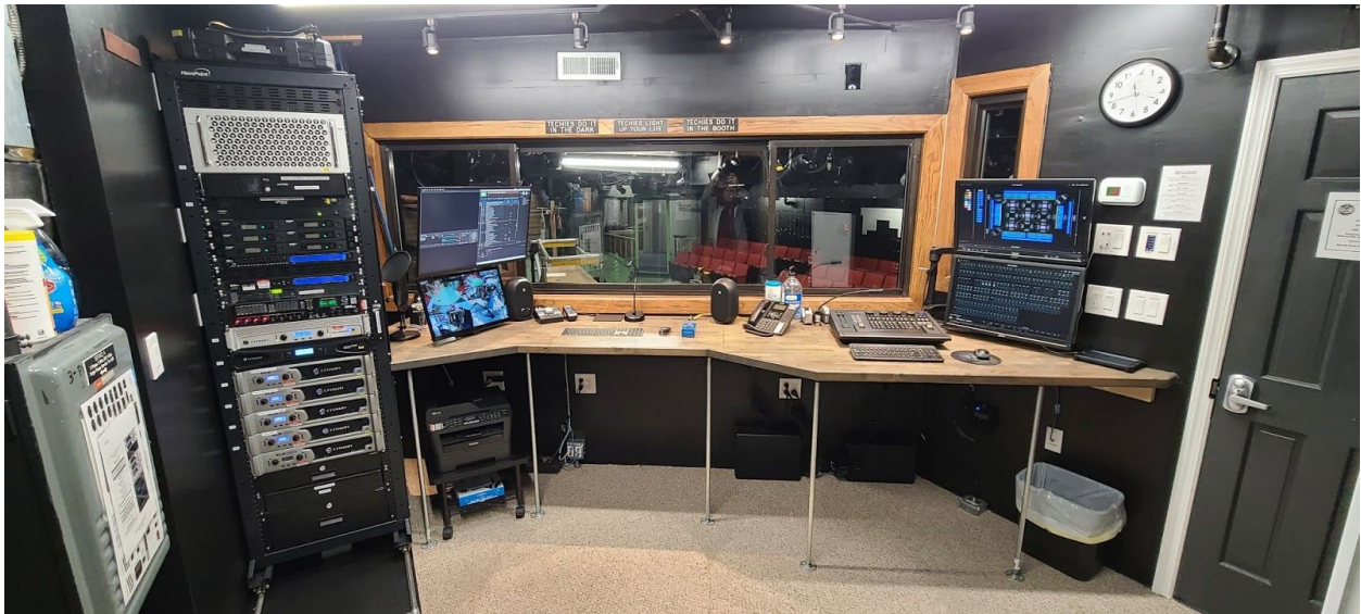
New Tech Booth layout showing new rack, desk, printer/cart, and floating monitors
