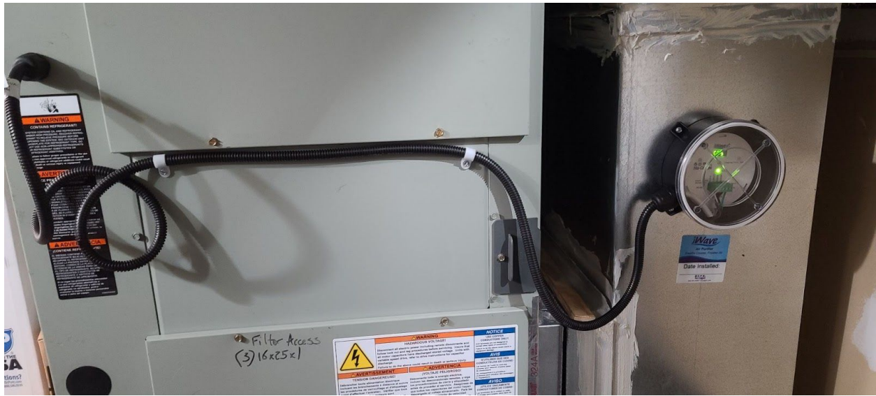
iWave Air Purifier installed on Lobby HVAC unit (round device on right)
