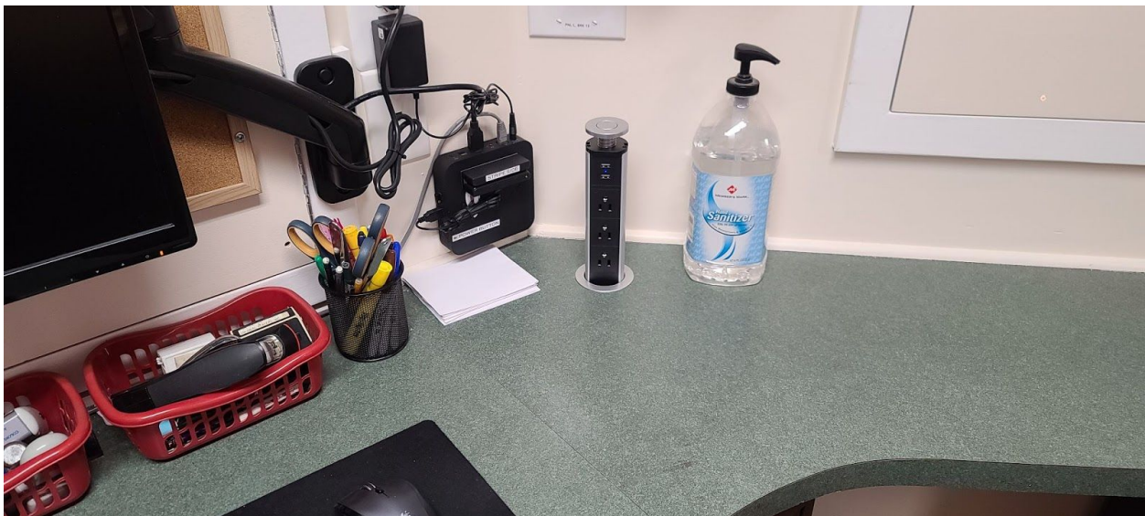
Pop-up power grommet with 3 outlets and 2 USB charging ports for volunteers
